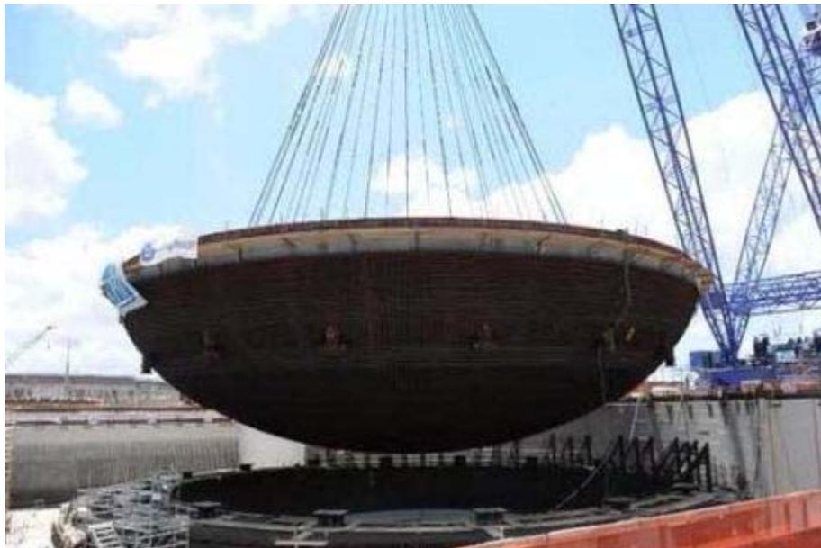
*The containment vessel bottom head is lowered onto its cradle (Image: Georgia Power)*
